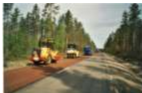
Y1B 8/11 = 12 kg ballast + 1,7 kg bitumen
