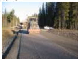
40 mm IMT 8/22 = 88 kg ballast + 3,6 kg bitumen
