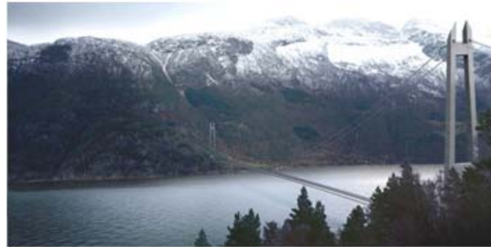
Hardangerbrua, 1310 m span, due to open in 2013
