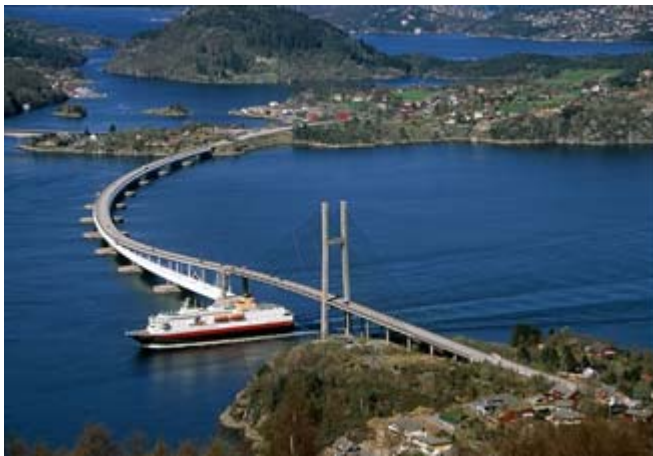
Nordhordalandsbrua, 1243 m floating span, opened in 1994
