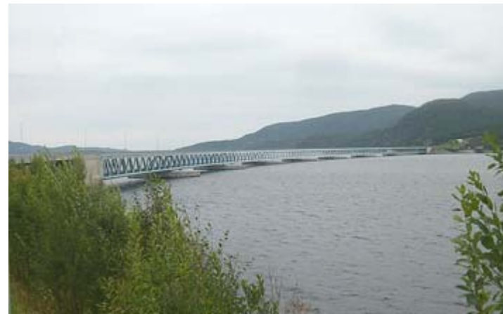
Bergsøysundbrua 931 m floating span, opened in 1992
