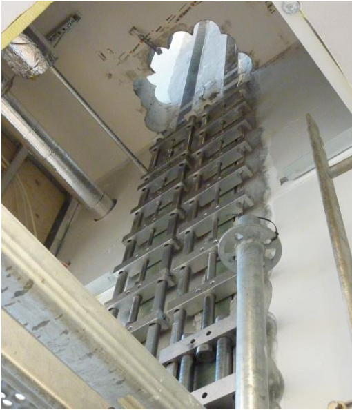
Strengthening of a structure using pre-stressed CFRP laminates in Umeå
